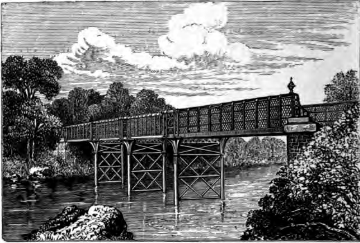
FIG. 72—THE PILMORE BRIDGE.
